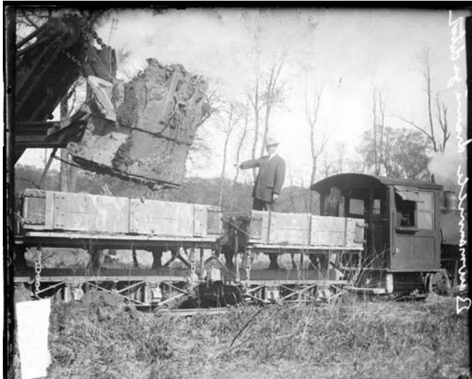
Loading Dirt Train at the North Shore Channel Near Bowmanville, 1909
